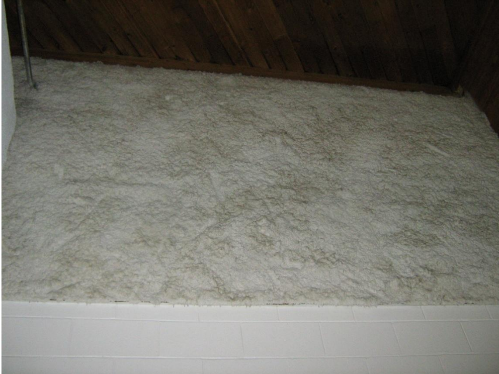
Photo 4: Non ACM blown fibrous insulation in Pool Area, (Rm. 237)
